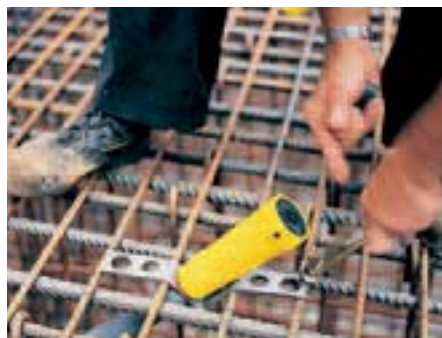
Anchor system is easily fixed to the reinforcement with wire and pliers.
