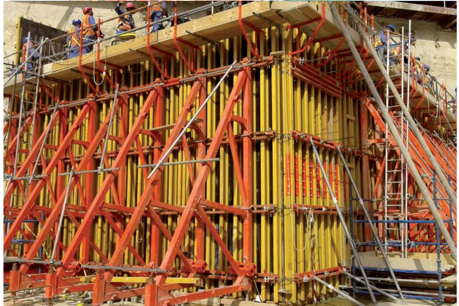
A Max. concreting height of 8.75 m, can be achieved using Brace Frame SB-A0, A, B and C with VARIO VT 20 wall formwork.
