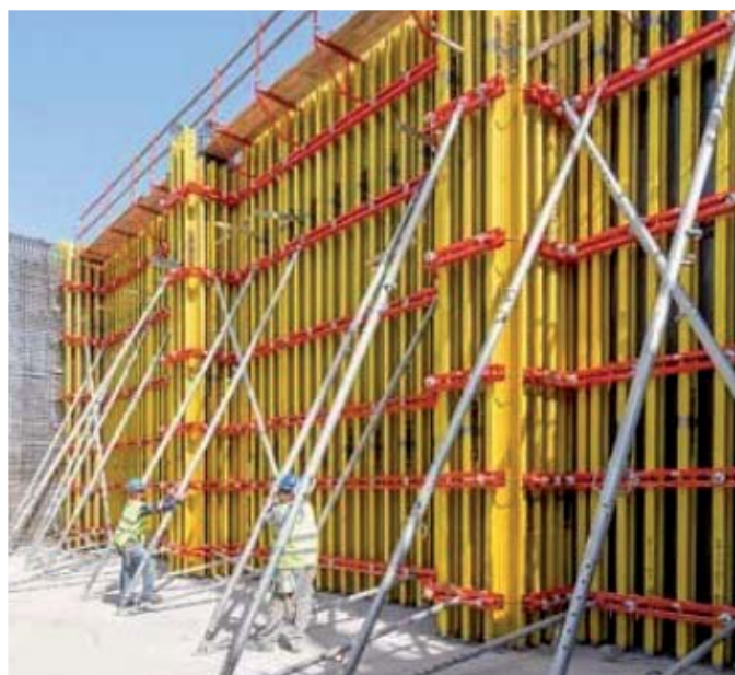
Extended VARIO VT 20 panels being used to shutter administration building.
