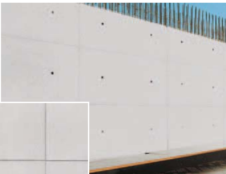
Perfect architectural concrete finish with horizontal and vertical panicular pattern.
