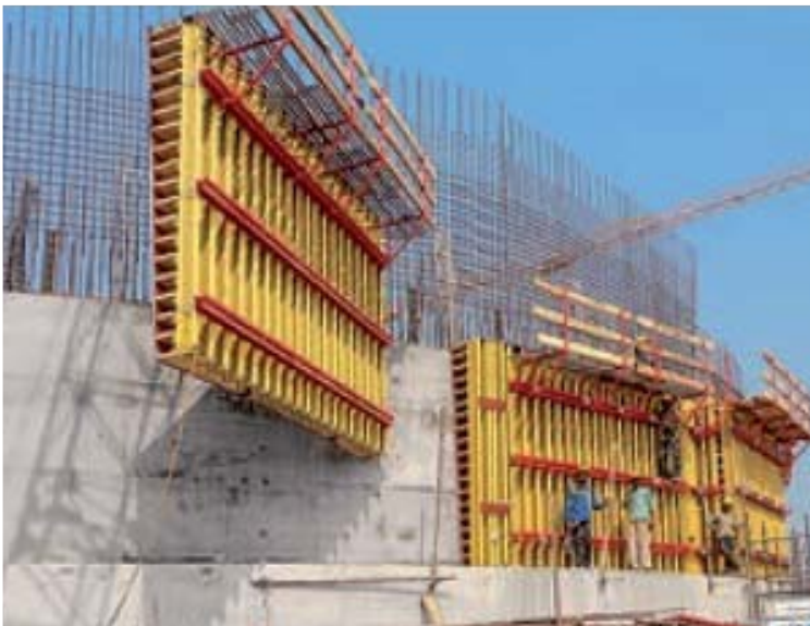
VARIO VT 20 being used to construct a circular tank. Timber on top of VT girders and steel walers produce the circular shape.
