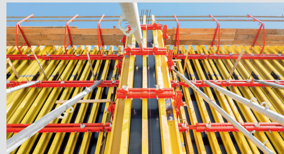
MULTIFLEX slab formwork with VT 20K girders. The use as main and secondary beams simplifies material requirements and planning.
