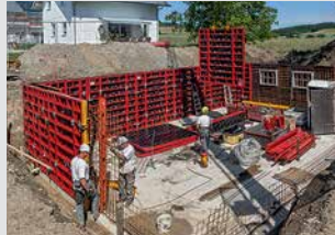
Wall Formwork
