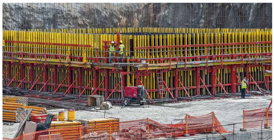
SCS system components are used for the vertical Starter with Brace Frames: Starter Bar SCS, Strongback SCS and the Heavy-Duty Spindle SCS.
