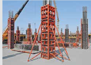
Column Formwork
