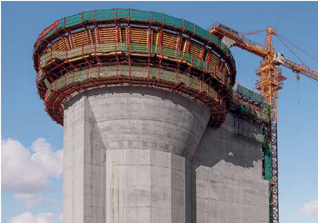
Free-form formwork on SCS Climbing Brackets for a large concrete funnel.
