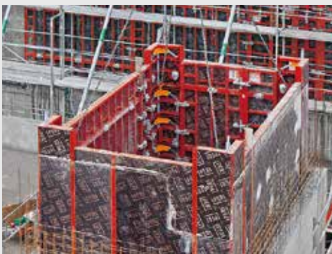
When releasing the shaft corners and pulling with the crane, a 35 mm striking clearance is created on each side.
