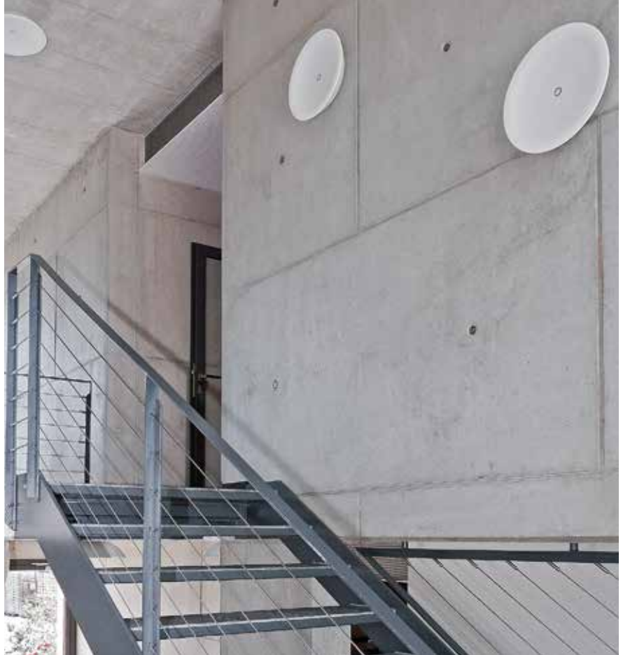
Walls that are formed using MAXIMO stand out due to the clean concrete finish of their surfaces. It is free from indentations, unused tie points and, consequently, bleeding through unsealed tie points.
