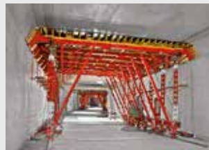
Tunnel Formwork
