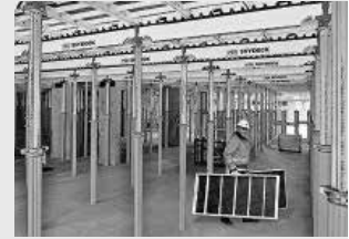
Slab Formwork
