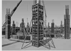
Column Formwork
