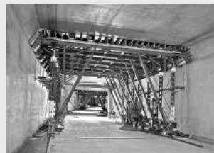
Tunnel Formwork
